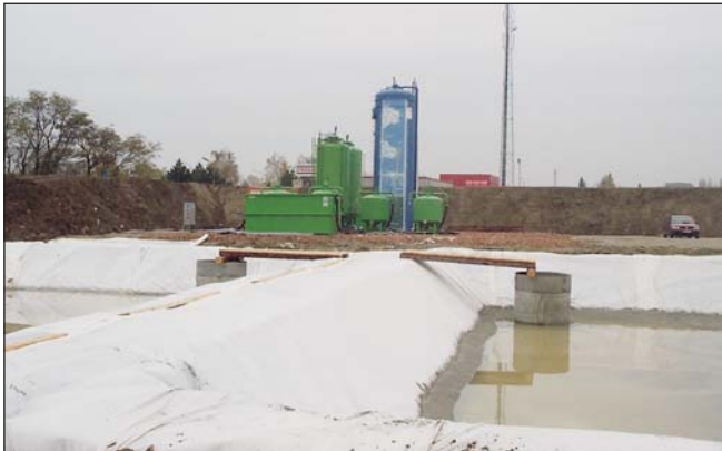
Sedimentation basins are made of special foil used for soil works.
