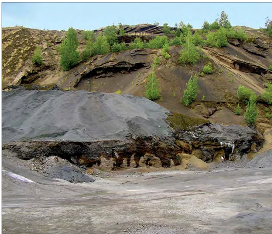
The leachate collected at the base of the slag heap contains cyanides and organic compounds. The adapted water treatment plant of BAUER Environment Group ensures a long term cost-saving and efficient treatment.
