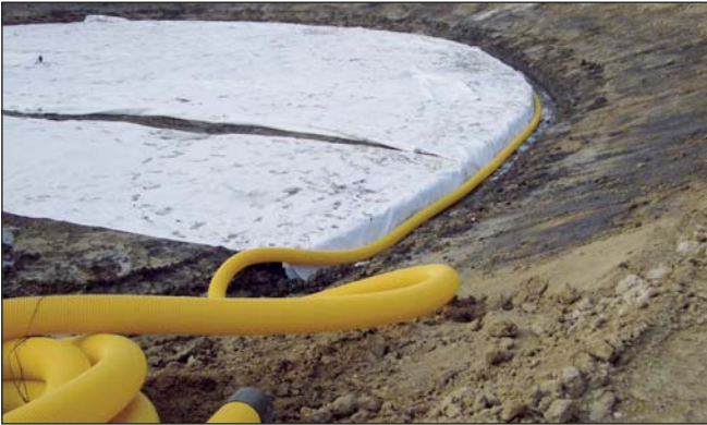
The filter body consists of a drainage layer (consisting of drainage pipes and drainage gravel) and a filter layer (drainage sand with a specific grain size distribution).
