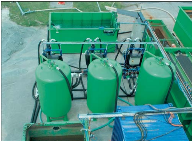
Fine particular matter and bound PAH are removed by the multi media filters. Consequently the lifespan of the activated carbon filters increases.
