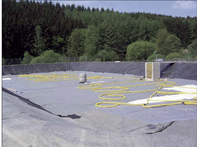
The drainage system for ventilation and drainage of sewage sludge has to be installed carefully to avoid damage of the sealing foil.
