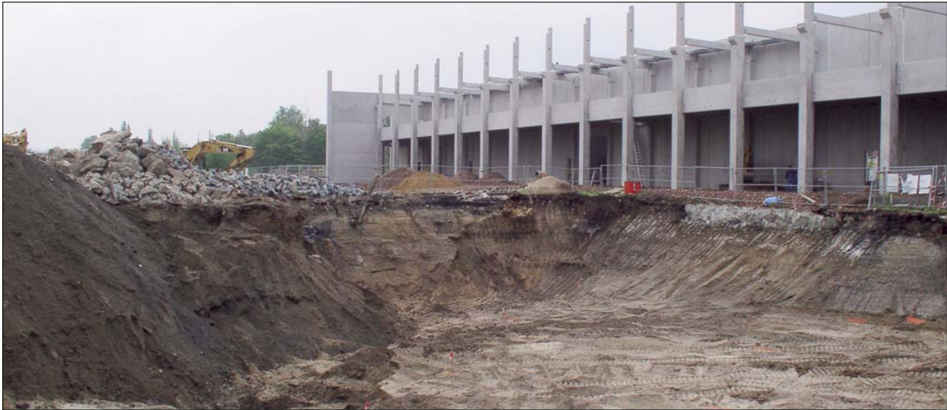
On the remediation site 173,000 to contaminated soil and 3,000 to contaminated construction waste had to be excavated and be disposed off.
