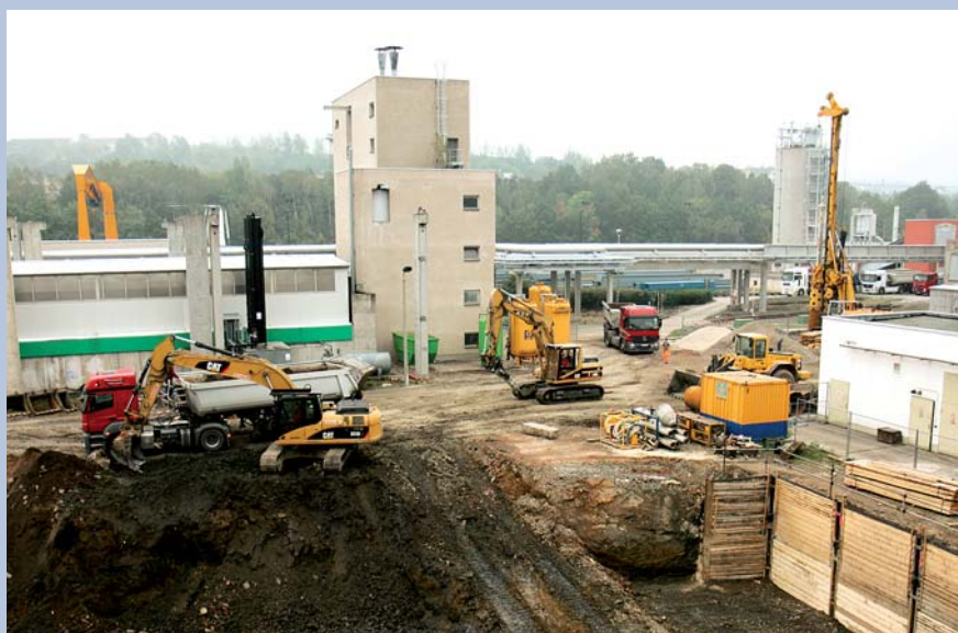
▲ The pits in Plauen had to be divided into multiple areas
