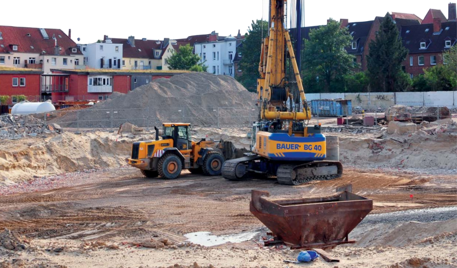
▲ Replacement bore drilling with a high-performance Bauer BG 40 rotary drilling rig
