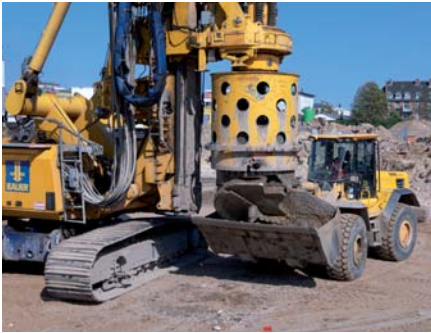
▲ Excavated material is sorted
